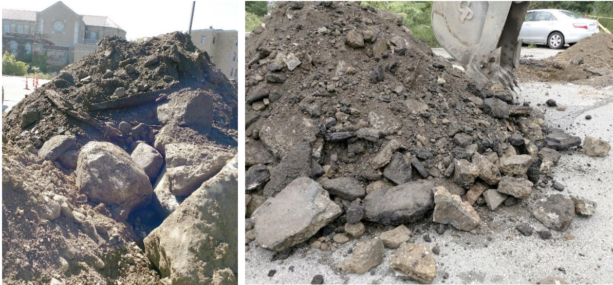
Figure 6. Fill encountered within Building 2 and 3 north of the 1955 fill line.
