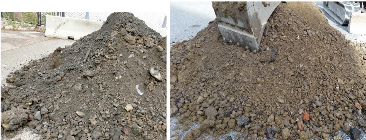
Figure 7. Fill encountered within footprints of Buildings 2 and 3 between 1938 and 1955 fill line.
