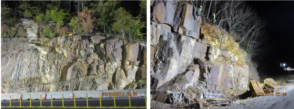
Figure 10 – Rock Slope Scaling at/near Area 9
