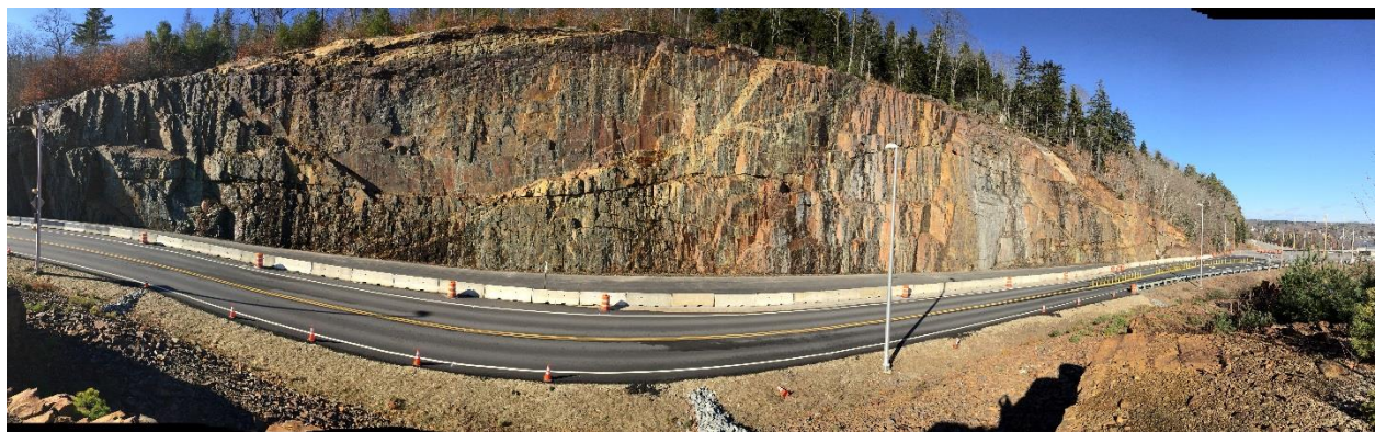
Figure 13 – Final Rock Slope Condition
