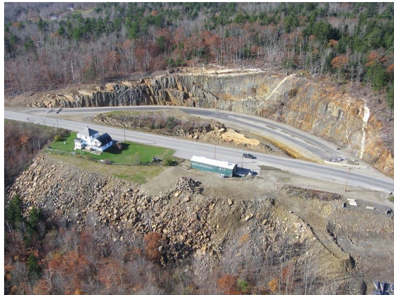
Figure 7 – Completed Rock Slope
