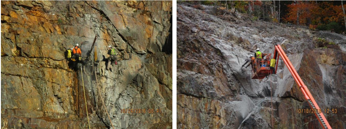
Figure 11 – Rock Dowel Drilling with Wagon Drill (left) and Manlift (right)
