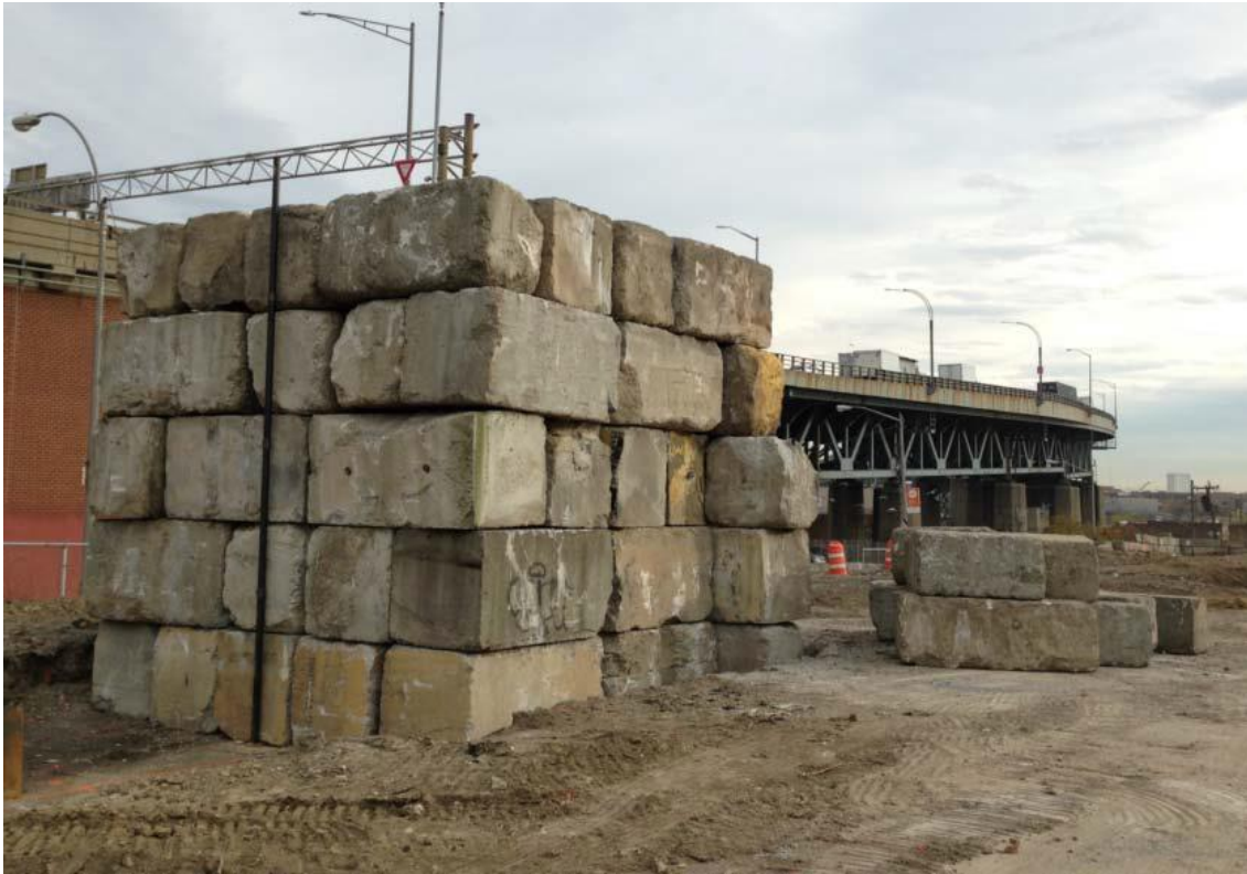
Figure 4. Settlement load test at the southeast corner of Varick Avenue
