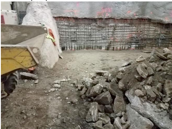
(10c) Installing Reinforcement Grid
