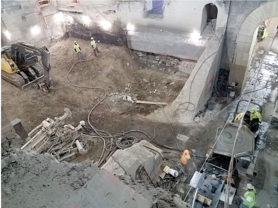
Figure 9. View of Support of Excavation Solution during Construction (image by Becker)
