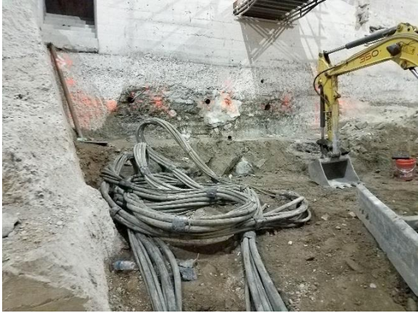
(10a) Bedrock Lift Excavation
