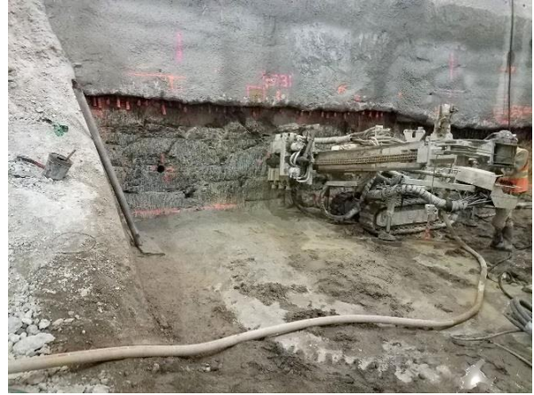
(10b) Drilling Rock Dowels
