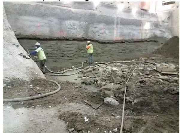
(10d) Shotcrete Wall
