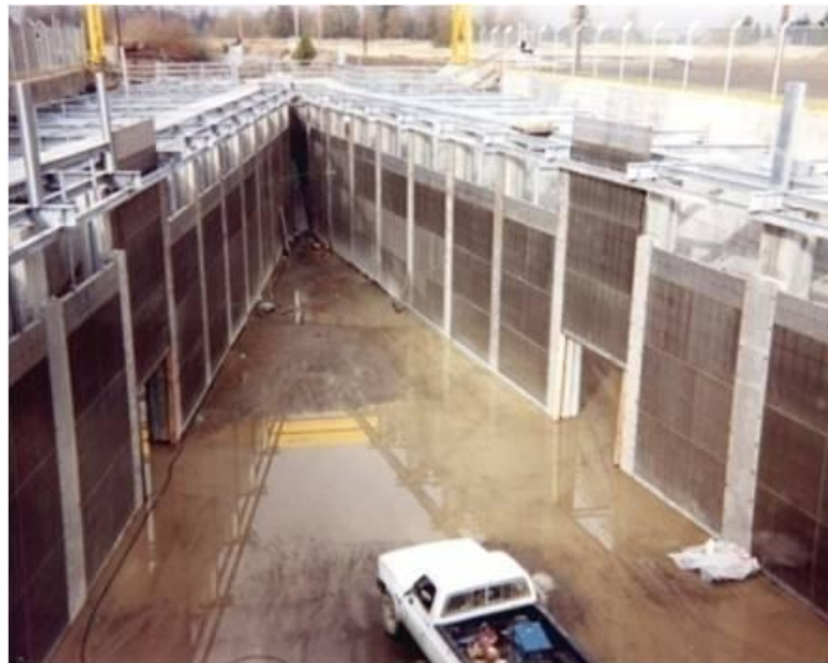
Figure 4 Angled screen diversion system (courtesy US Filter)
