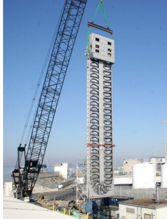
Figure 7 Passavant Geiger MultiDsic travelling water screen (courtesy Alden Research Laboratory)
