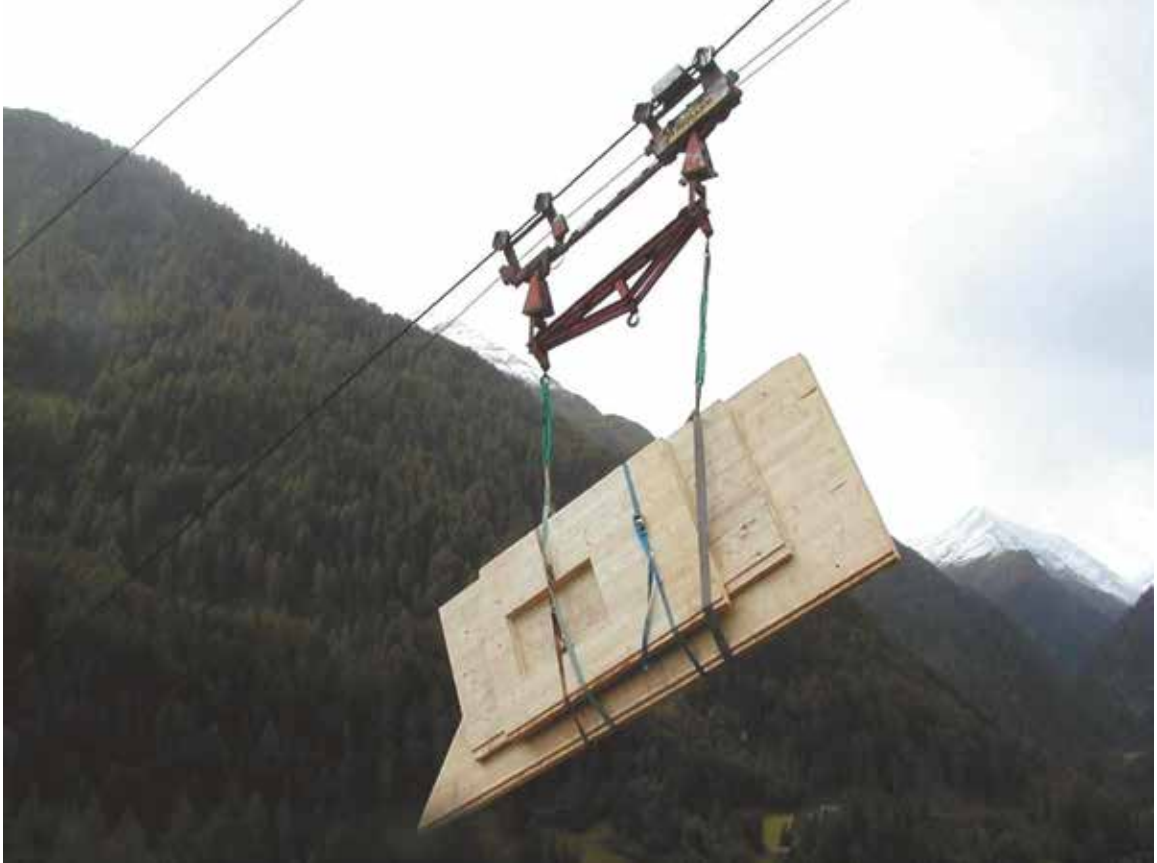
Figure 2 Lifting and handling of CLT elements by cableway (courtesy of KLH)
