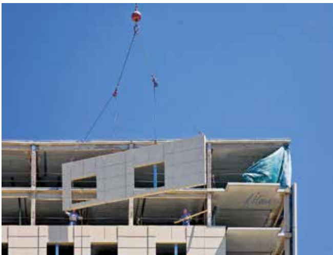
Figure 1 Lifting and handling of precast concrete elements
