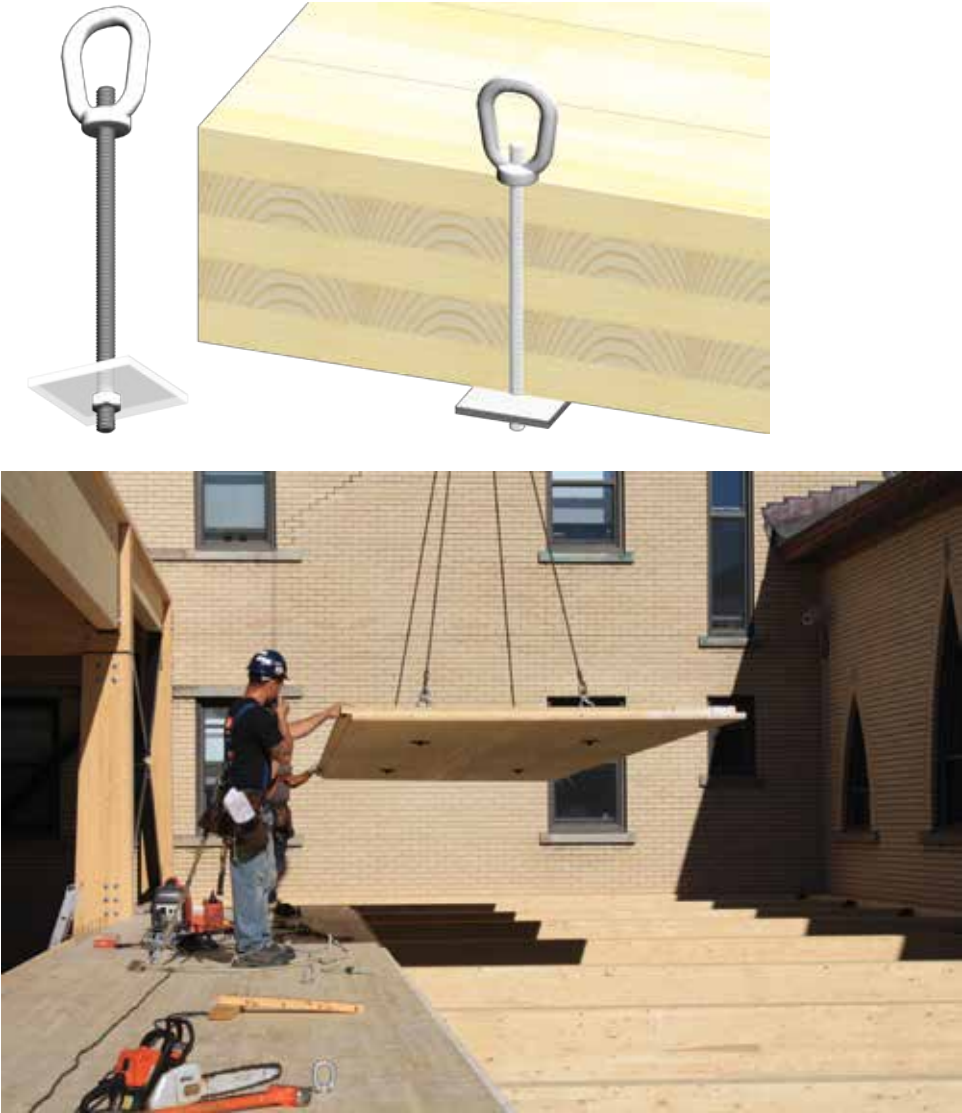
Figure 17 Eyelet used with threaded bolt or sleeve and steel plate (courtesy of Nordic Engineered Wood)
