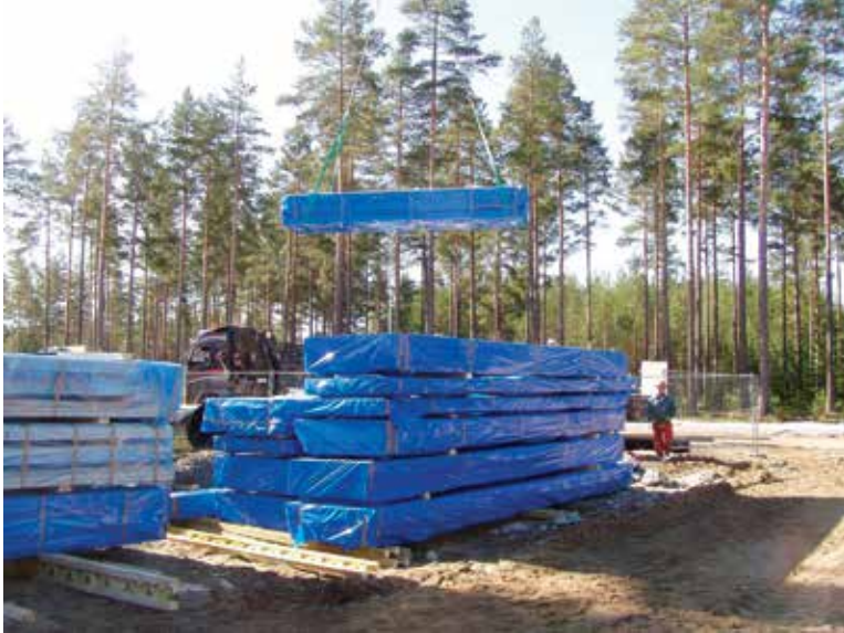
Figure 55 Storage on construction site – individually wrapped bundles stacked on lumber skids
