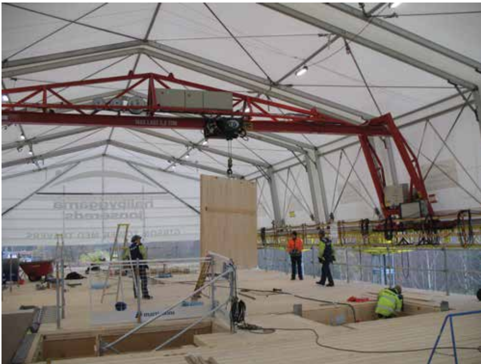
Figure 9 Lifting and handling of CLT elements, in Sweden
