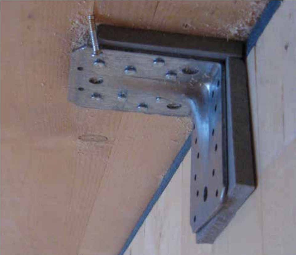
Figure 41 Sealing joint between floor, wall, and connectors
