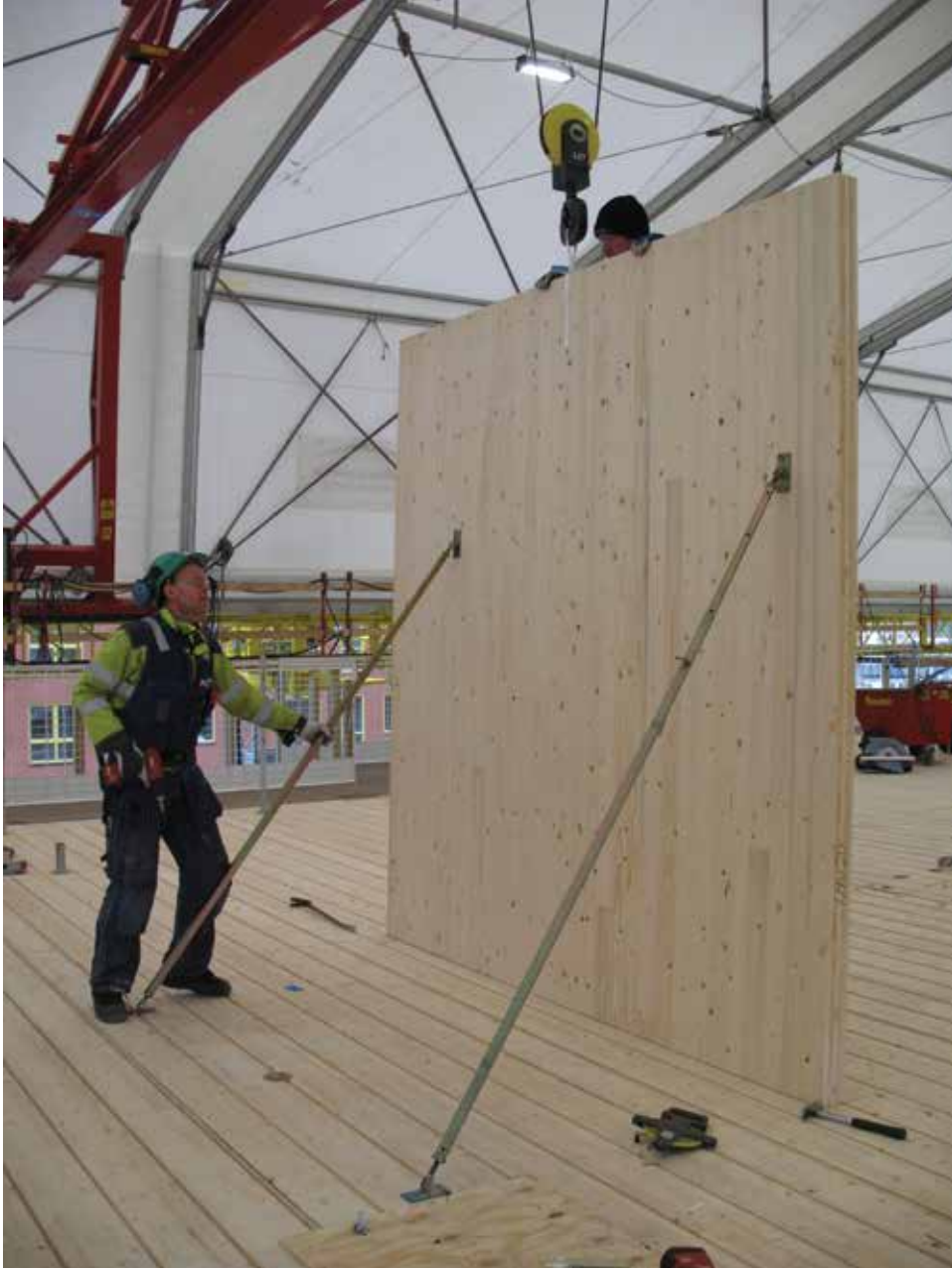
Figure 44 Adjustable shoring for walls
