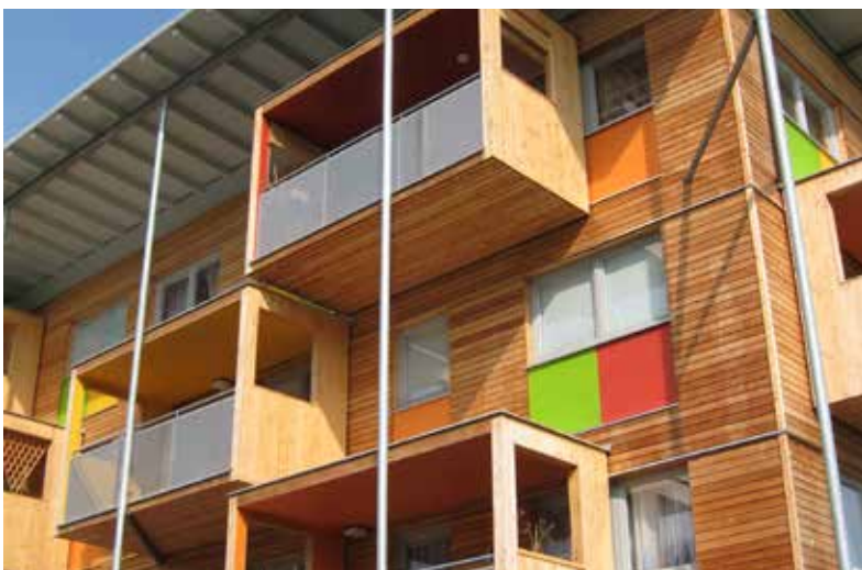
Figure 19 Multi-family building in Judenburg, Austria (courtesy of KLH)
