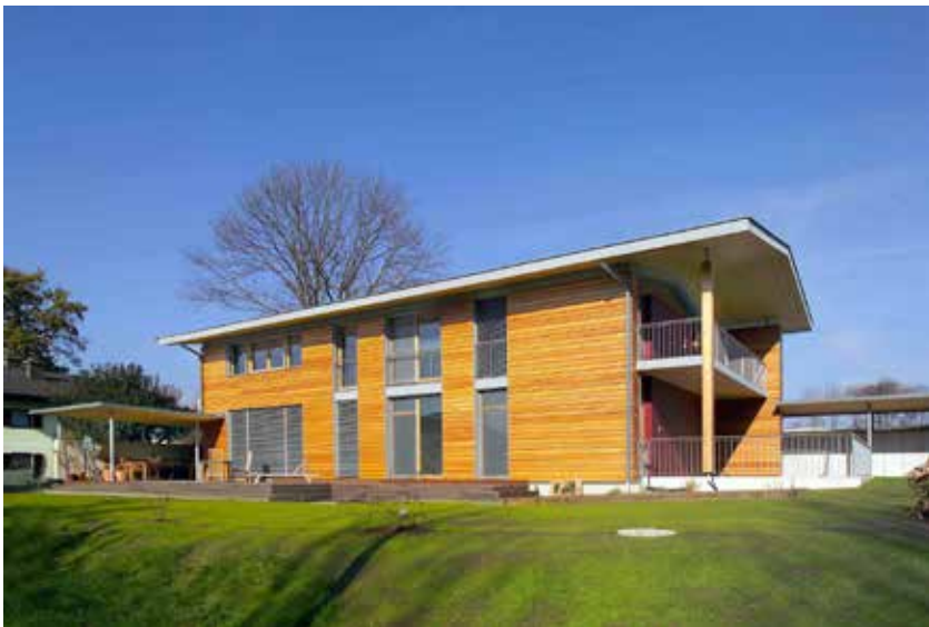
Figure 16 Single-family house in Klagenfurt, Austria (courtesy of KLH)
