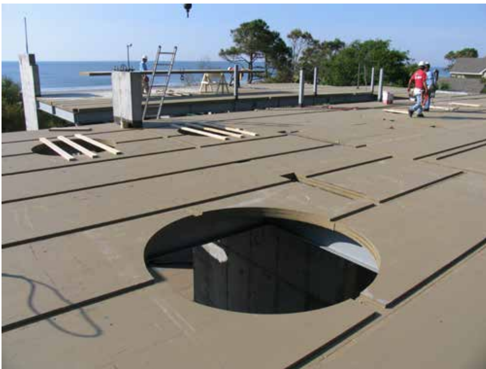
Figure 31 Residential building in South Carolina, United States (courtesy of Binderholz)
