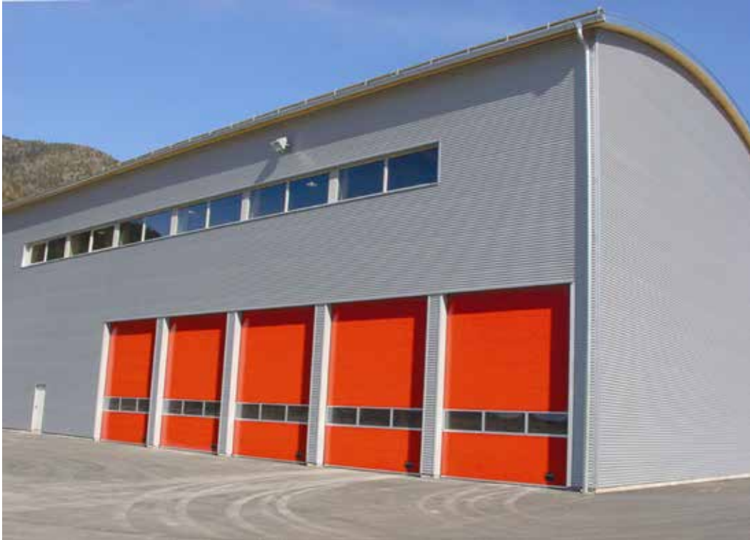
Figure 29 Kommissionshalle, Katsch, Austria (courtesy of KLH)
