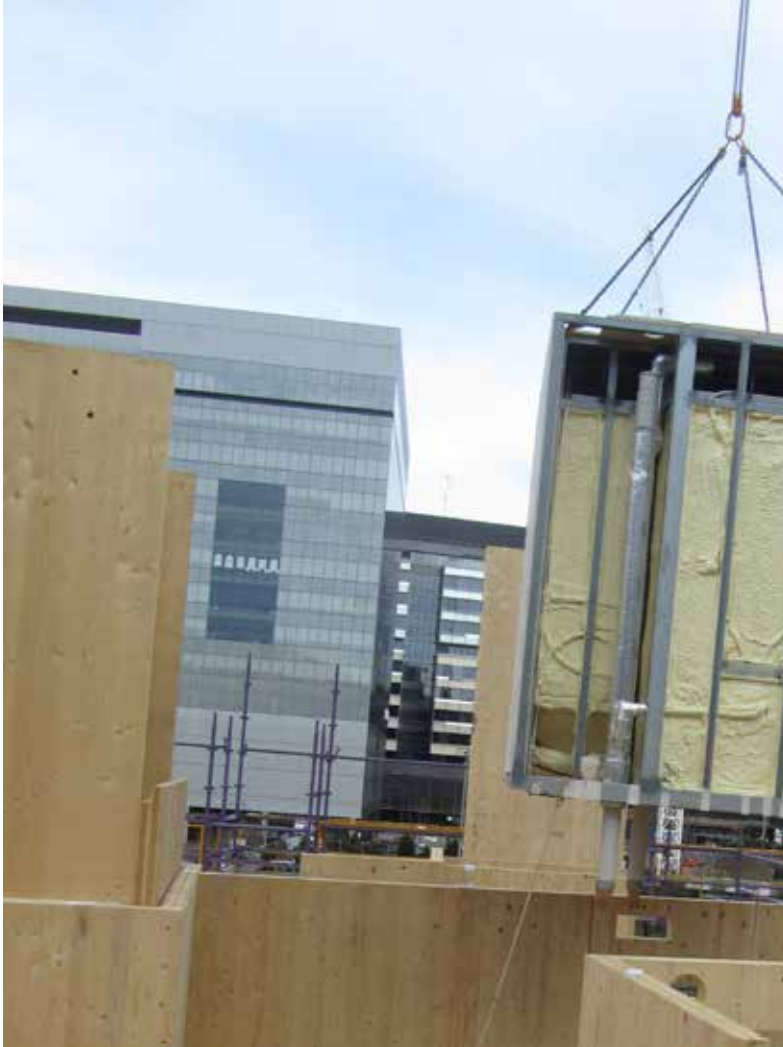
Figure 23 10-story apartment building in Australia (courtesy of Lend Lease, www.forteliving.com.au )
