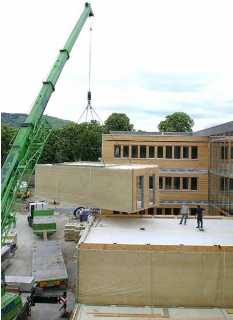
Figure 24 Impulsezentrum, Graz, Austria (courtesy of KLH)
