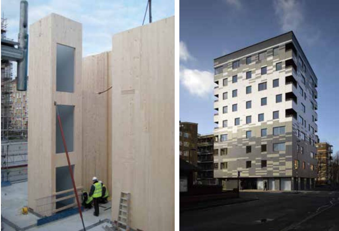
Figure 1 Typical CLT panel, typical CLT construction and a rendering of the 9-story CLT building in England
