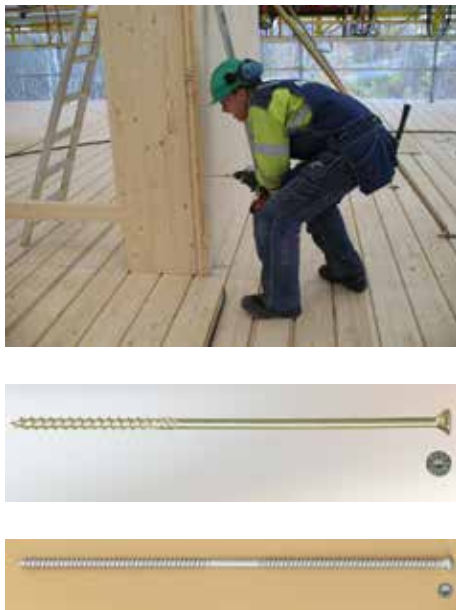
Figure 3 Self-tapping screws used in CLT connections
