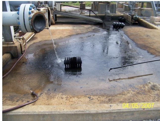
Figure 3 Use water to clean pigs removed from receiver whenever pyrophoric iron is suspected.
