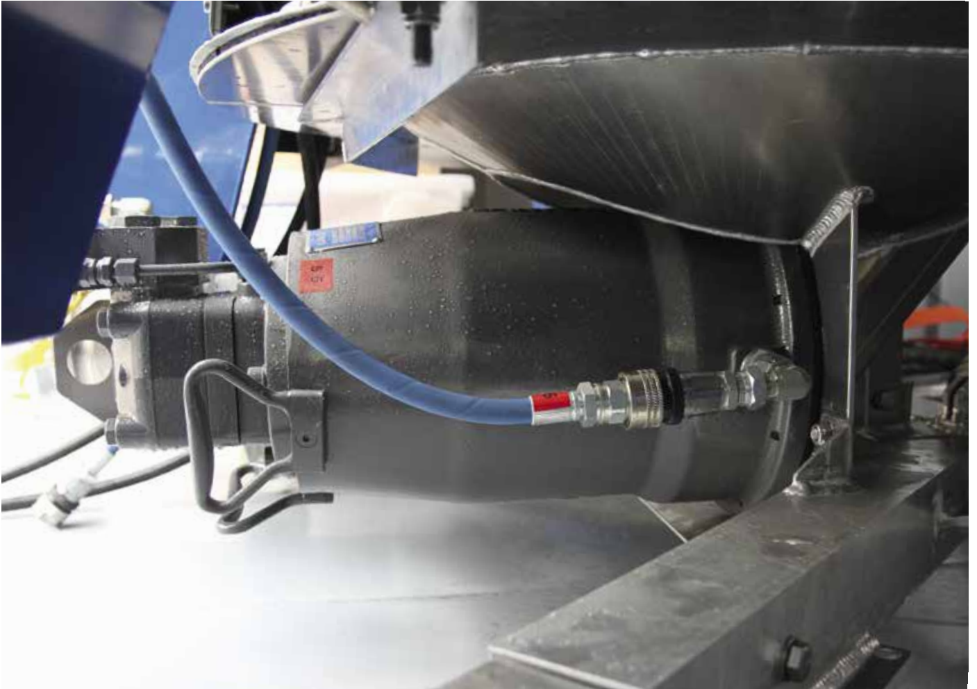
Hot water injection to pump
