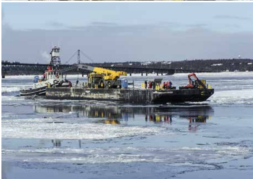
Marine Pollution Control (MPC) was awarded a contract by the USCG Research and Development Center to provide specific equipment suites to facilitate the 'Oil in Ice' demonstration.
