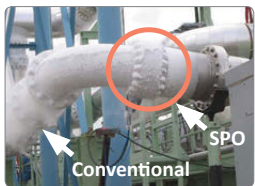
Cryogenic applications Leaking conventional flanges vs. leakfree Vector SPO® Compact Flange.
