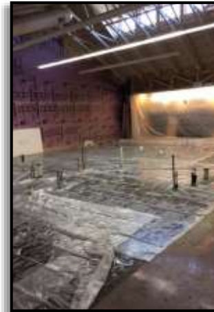
Underground Rough Ins
