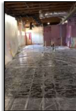
Concrete Poured in Phase 6
