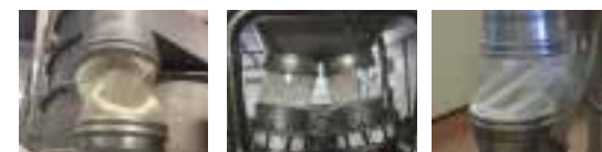
Installation gap too small Installation gap optimal Installation gap too large
