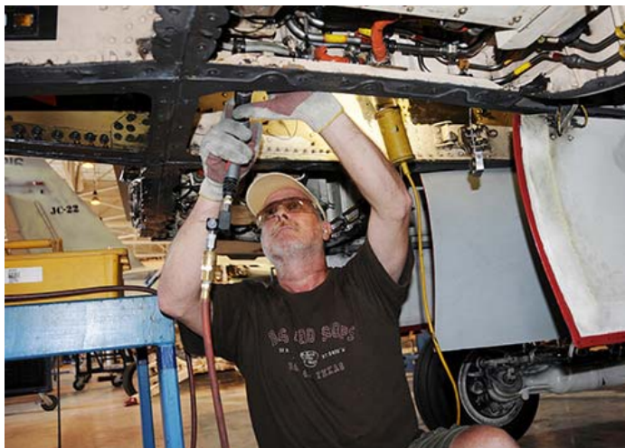
Kai Boyce, an aircraft artisan at FRC Southeast in Jacksonville, Fla., makes a repair in the auxiliary power unit compartment of an F/A-18 Hornet in June. (Photo by Victor Pitts)
