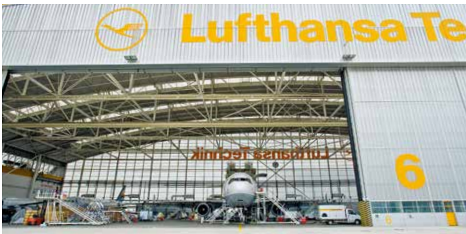
The hangar of Lufthansa Technik Maintenance International in Frankfurt.
