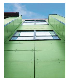
Synapse Construction built 3D models and came up with several iterations of what the siding would look like. The homeowner opted for Trespa Pura NFC flush siding (in Royal Mahogany) paired with olive-treated Silbonit panels for a striking mix of exterior materials. The company merged downspouts whenever possible and tucked them into less noticeable corners to limit the amount of piping on the facade.
