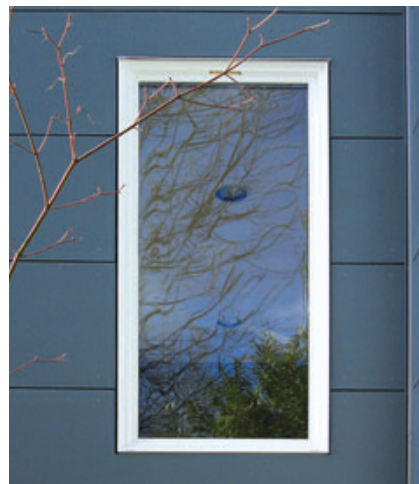
Figure 6. The architect specified a trimless window design, in which both the cedar siding and the fiber-cement panels stopped short of the exposed frames, leaving a reveal that matches those between courses.
