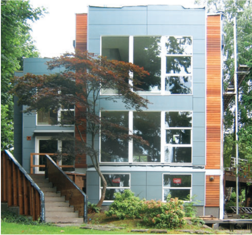
Figure 1. The open-joint method can be used with either board or panel siding. While most often used in commercial construction, it's gaining popularity in residential applications, too.
