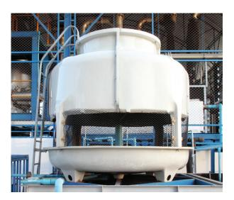
TOWER TABS Scale & Corrosion Control Tablets treatment requires no supplemental pH control and it protects ferrous and non-ferrous metals while inhibiting the formation of hard mineral scale in high hardness, high alkalinity makeup water. This product contains soluble zinc as an active ingredient, which is also a tracer to track precise treatment doses in the field.
