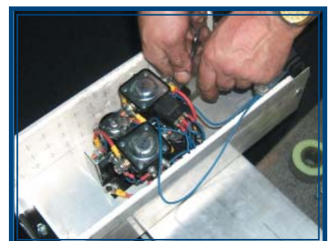
Pic E - F: Install New Solenoid
