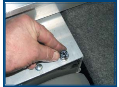
Pic L - C: Re-install Fuse and test
