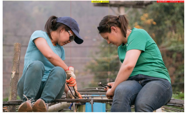
VINNIE detecting people missing hard hats and safety vests. (Photo courtesy of ENR)
