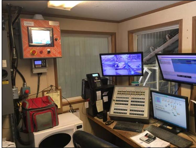
**Figure 2:** HMI/PLC enclosure (top left) mounted in customer batch office.
