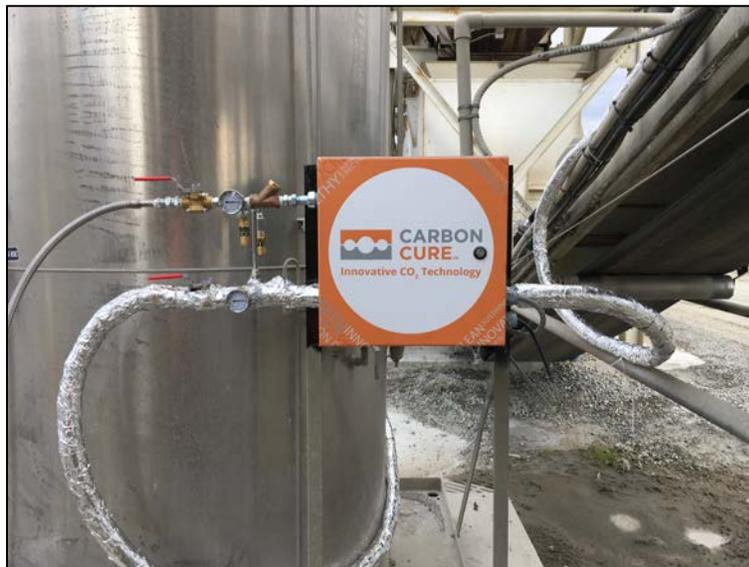
**Figure 1:** Valve enclosure mounted next to CO<sub>2</sub> supply vessel.
