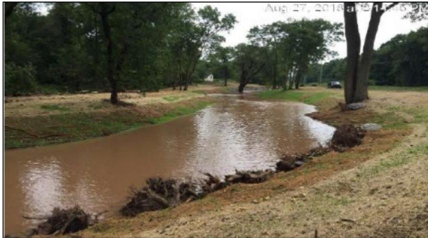
Streambank projects were carefully planned to reduce erosion and provide habitat. **Outagamie County placed toe wood structures at the base of this restoration project.**
