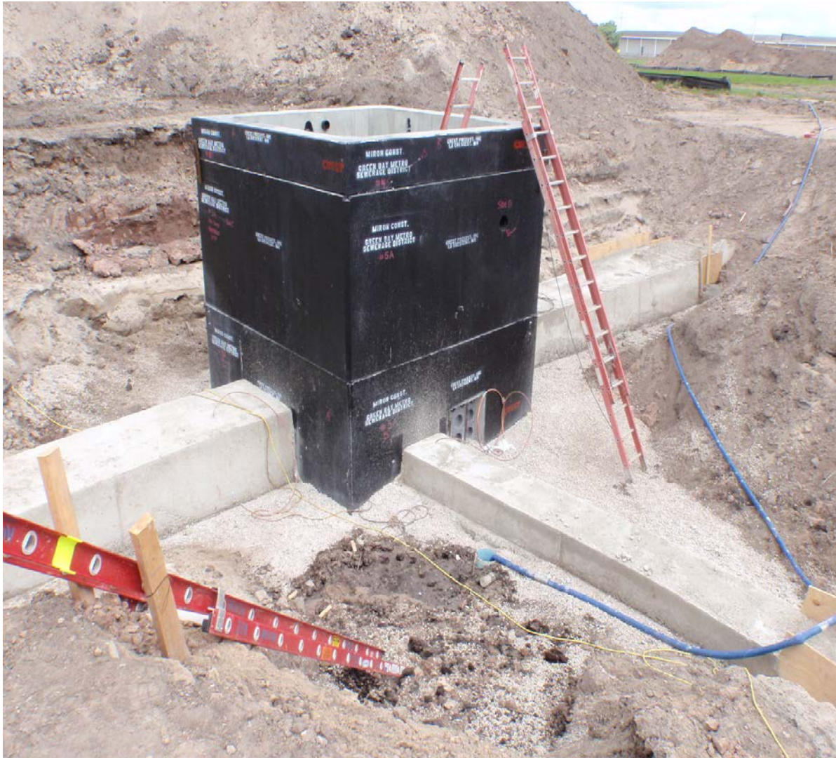
Completed Duct Banks X, Y, and C at EMH-5A
