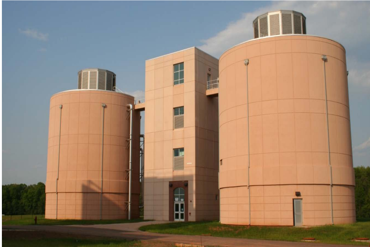
Silo-Shaped Digesters at Broad Run WRF in Loudoun County, VA, USA
