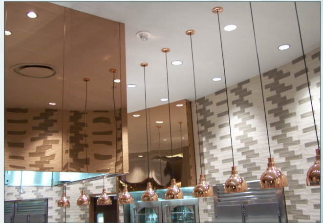
Mirrored copper hoods with matching lighting
