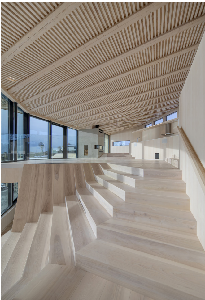
A floating roof covers the whole structure, only held up by the facades and ridge beam.
