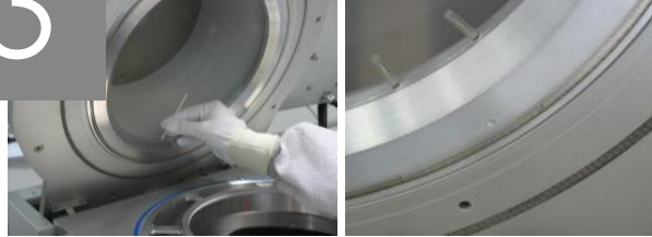
Installation of the 24 quartz tubes in liner's holes
