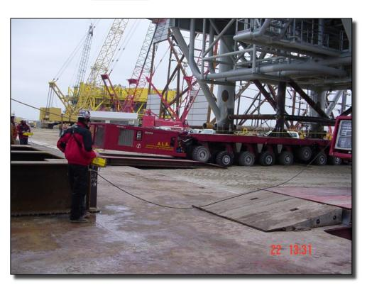
The C-DECK load out actually went smooth, just a flat tire on each of the transporters that needed to be isolated.
