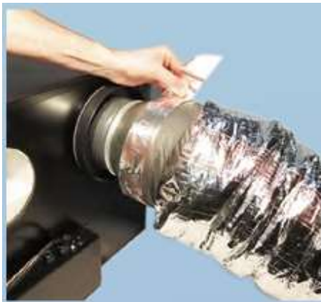
3. Tape Inner Duct
