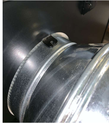
2. Apply sealant, insert duct, and run fastening screws in place
