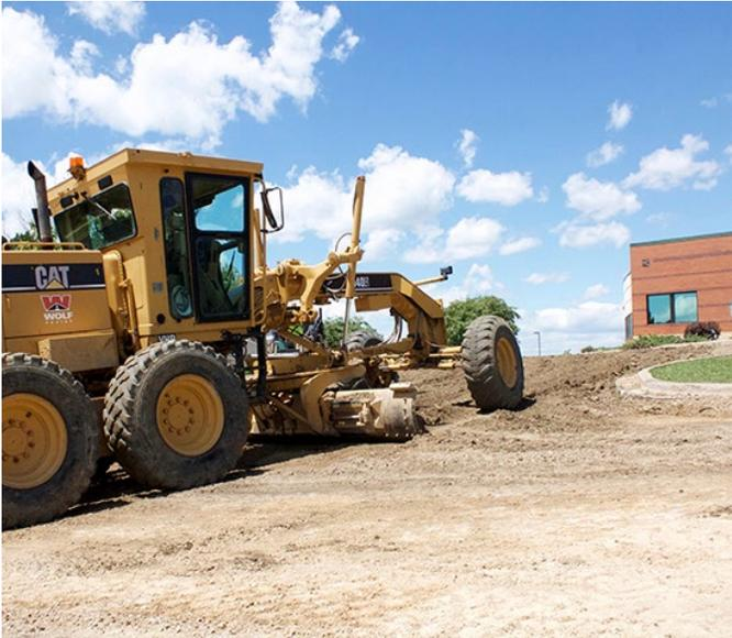
**Fine grading** – grading is completed to manage water run-off appropriately. During the proof row of this project, the Wolf Paving team came across unforeseen soft clay areas in the sub base that required repair. To manage this additional cost, Wolf Paving used a new technique called plowing to undercut the sub base and mix the soft clay with aggregate to improve the strength of the compromised areas.
